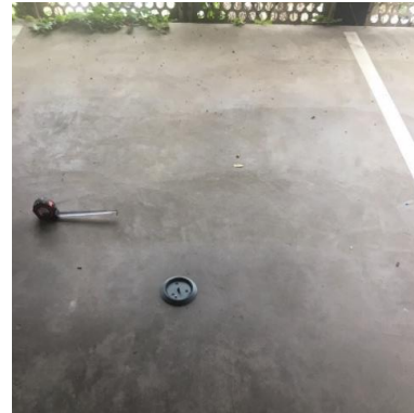
Figure 13 Sensor base installed
