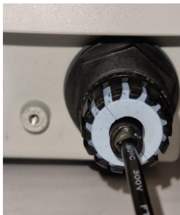
Figure 8: View of the rubber placement
