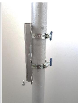
Installation support on a pole with strapping
