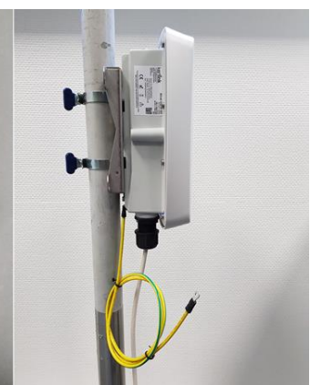
Installation the Wirnet™ iStation on the support
